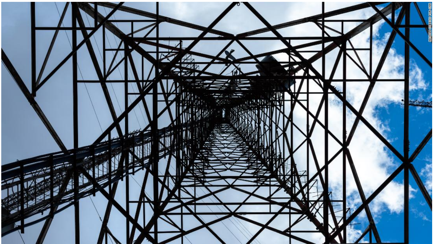
A StarTimes transmission site in Limuru, Kenya.
